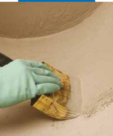
Waterproofing of details by brush
