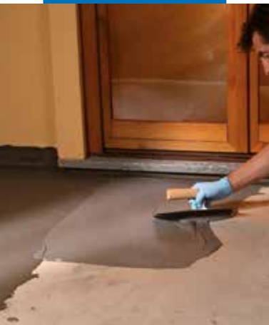
Waterproofing of terraces by trowel
