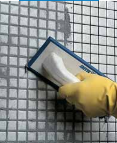
Grouting a glass mosaic (bathroom) with a float
